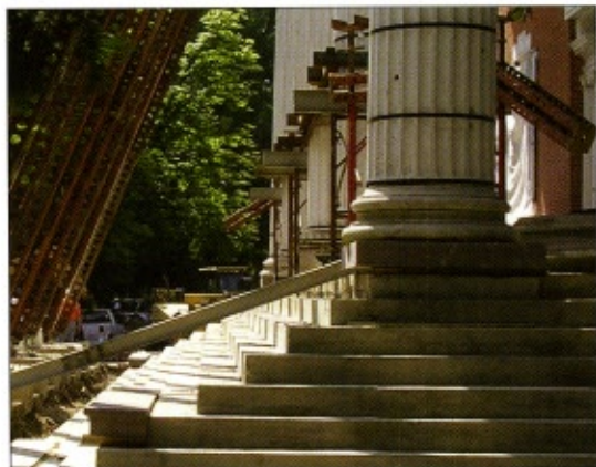
Mead Hall steps under construction
